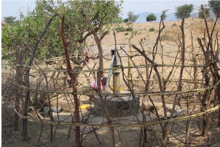
Figure 5.13: Shallow borehole with hand pump in Isinde Street, Tunduma TC (Source: TDA Field Data – Jumanne Placid)
